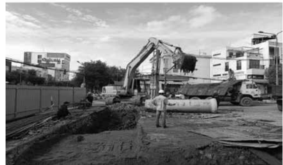
Figure 2. Upgrading of Tran Van Hoai Street (Photo taken on February 24, 2025)
